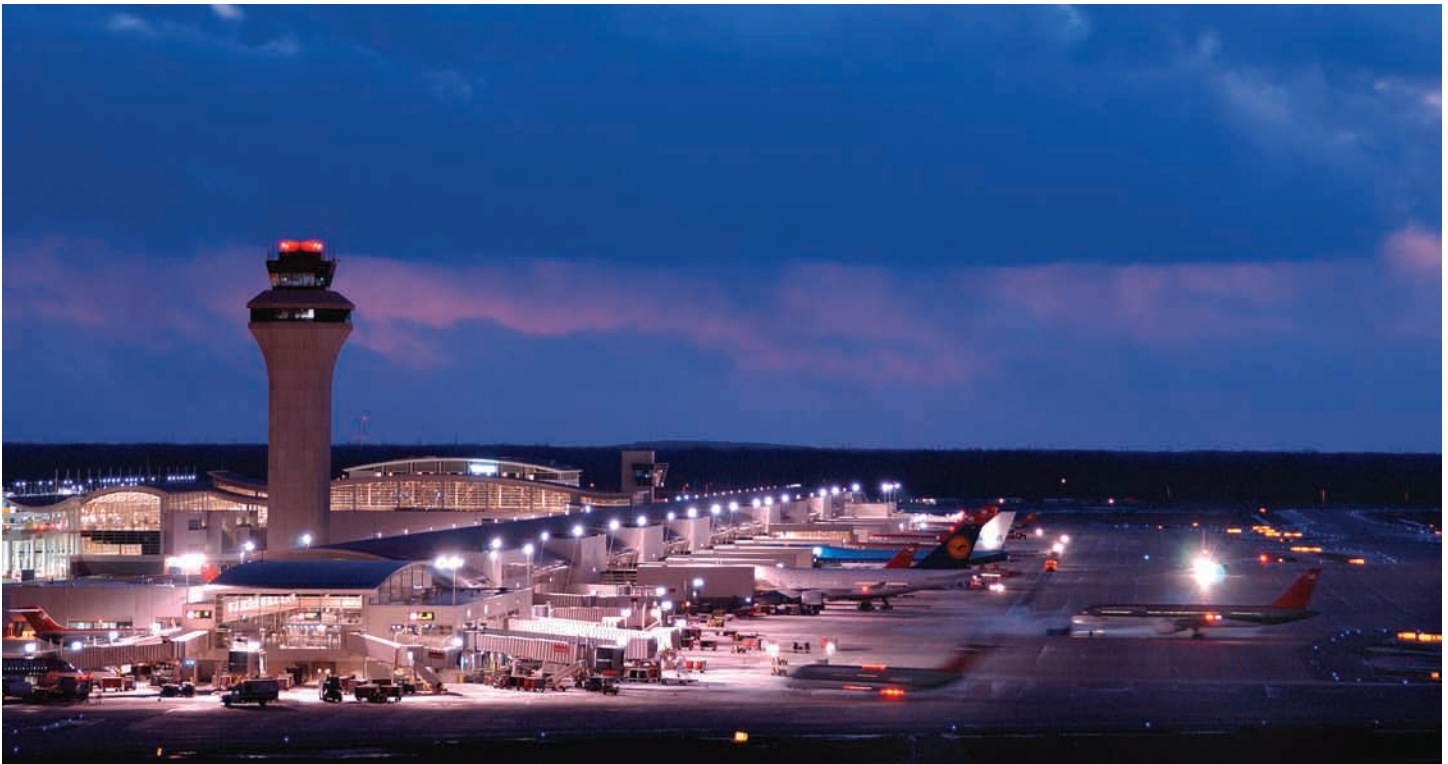
Detroit Metro Wayne County Airport is turning into an aerotropolis. Those woods in the distance will disappear. In their place will rise distribution centers, hotels, and other job-creators—the centerpiece, Kasarda says, of Detroit’s long-awaited revival. Photo courtesy of Aerotropolis Development Corporation.
