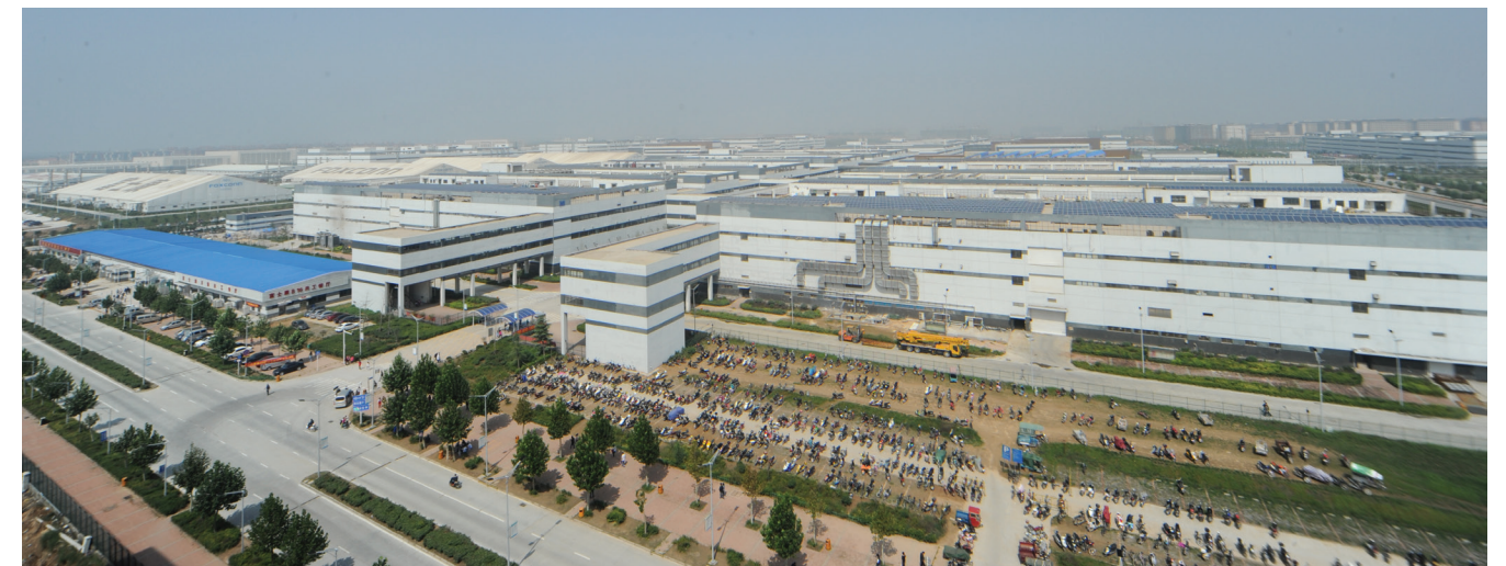
Foxconn's ZAEZ complex, which employs about 250,000, manufactures most of the world's Apple iPhones. Photo courtesy of ZAEZ
